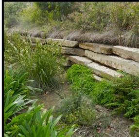
**3. Seep**—This wall of stacked limestone serves as a barrier that keeps stormwater from the lawns and parking lot from rushing into the swale below. Instead, the water slowly trickles out joints in the wall for days after a rain. The seep's micro climate supports shade and moisture-loving plants such as Maidenhair Fern, Wood Fern, Spider Lily, Buttonbush, and Spicebush.
